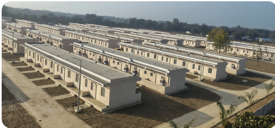
Phase 5 Housing: International-standard township housing
